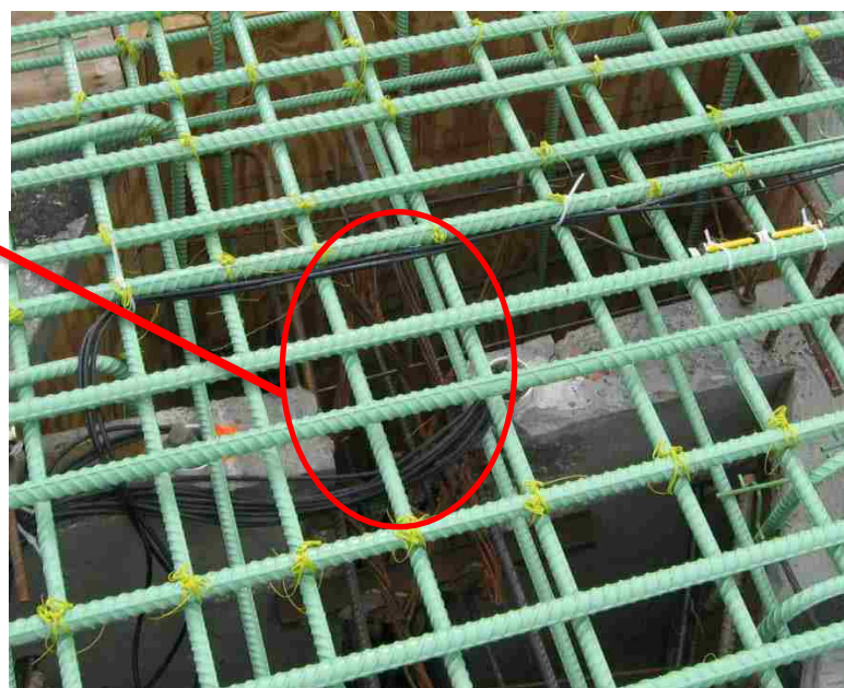
Figure 2.14 Intermediate bent in highway-50 Bridge with top strands highlighted
