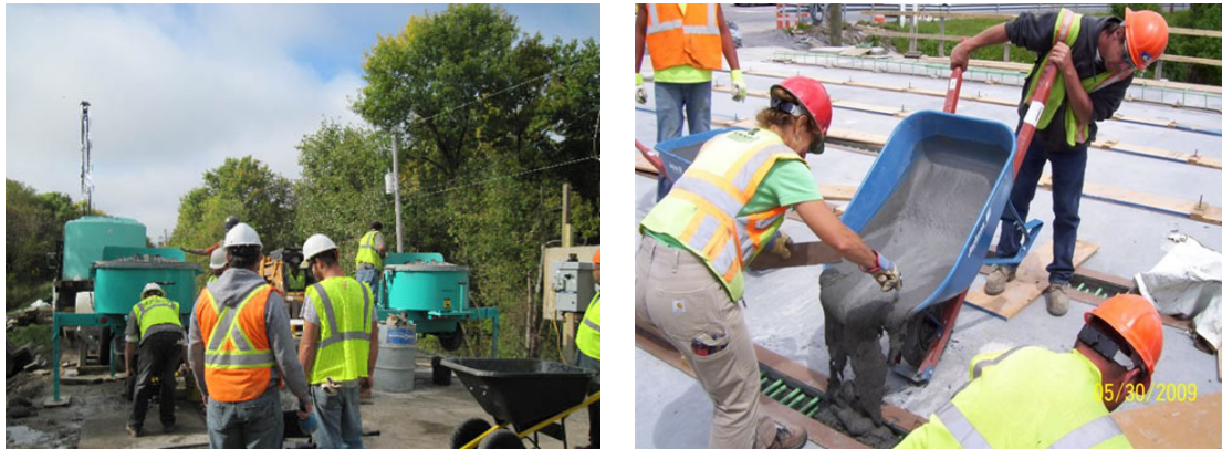
Figure 2.2 Batching and casting UHPC at site (FHWA, 2016)
