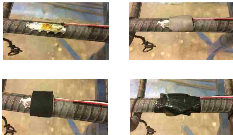
Figure 5.10 Strain gauge installation
