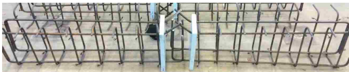
Figure 3.9 Reinforcement layout with joint detail
